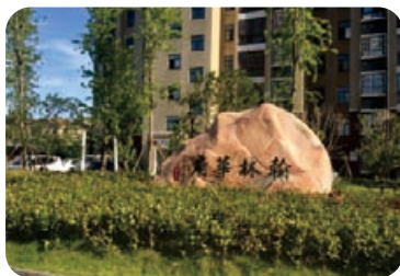
内蒙古赤峰市翰林华府 Hanlin Huafu Residential Area in Chifeng, Inner Mongolia Province
