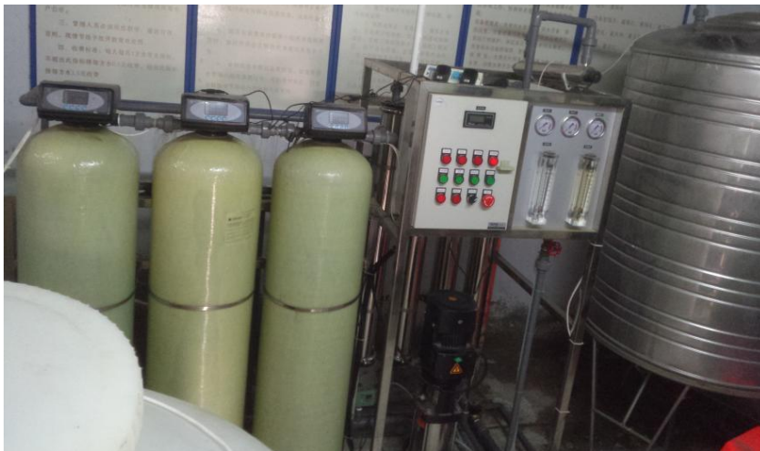
Figure 1-15 RO pre-treatment system
