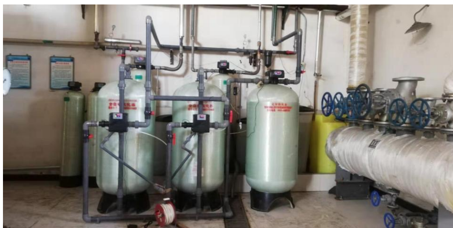
Figure 1-24 Deoxygenation system
