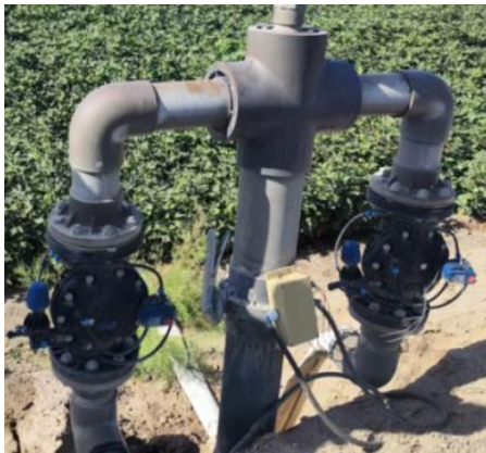
Figure 2-22: One water outlet pile connected to two diaphragm valves
