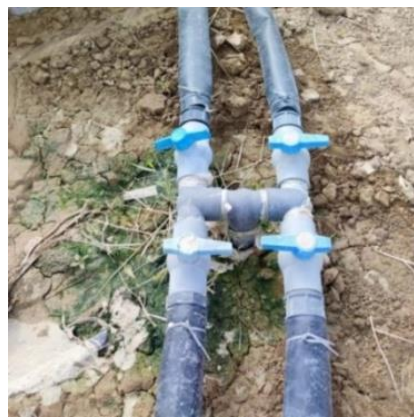
Figure 2-23: One water outlet pile connected to four ball valves
