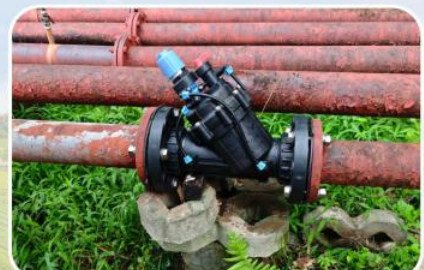
◎浙江温州某高尔夫球场 (DN100减压阀) Wenzhou, Zhejiang – Golf Course (DN100 pressure reducing valve)
