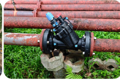
◎浙江温州某高尔夫球场 (DN100减压阀) Wenzhou, Zhejiang – Golf Course (DN100 pressure reducing valve)
