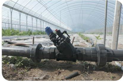
◎浙江温州山福镇某无花果种植园 (DN65减压阀/持压阀) Wenzhou, Zhejiang – Shanfu Town Fig Orchard (DN65 pressure reducing/pressure sustaining valve)
