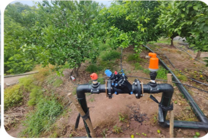
◎四川资阳某150亩柑橘种植园 (DN80减压阀) Ziyang, Sichuan – 100,000 m 2 Citrus Orchard (DN80 pressure reducing valve)
